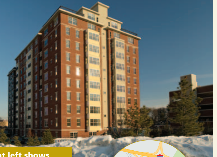
The rendition at left shows Avalon Natick's layout. The photo above shows one of the buildings near the end of construction in Feb. 2013.
